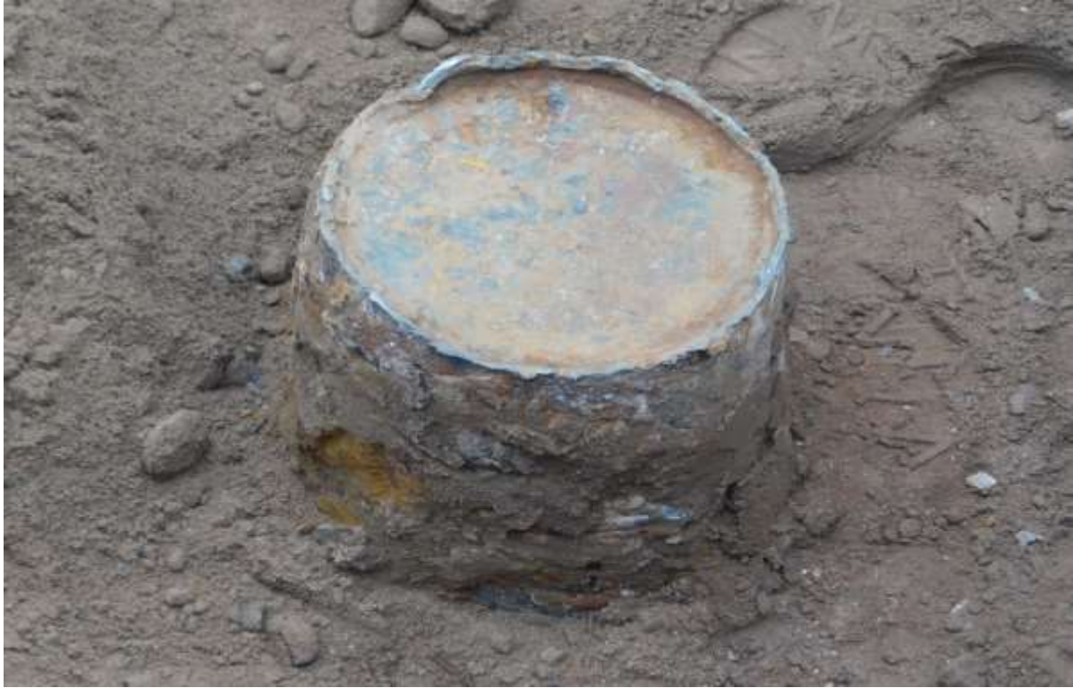
9. Close-up photo of cleaned top of well casing in excavation pit.
