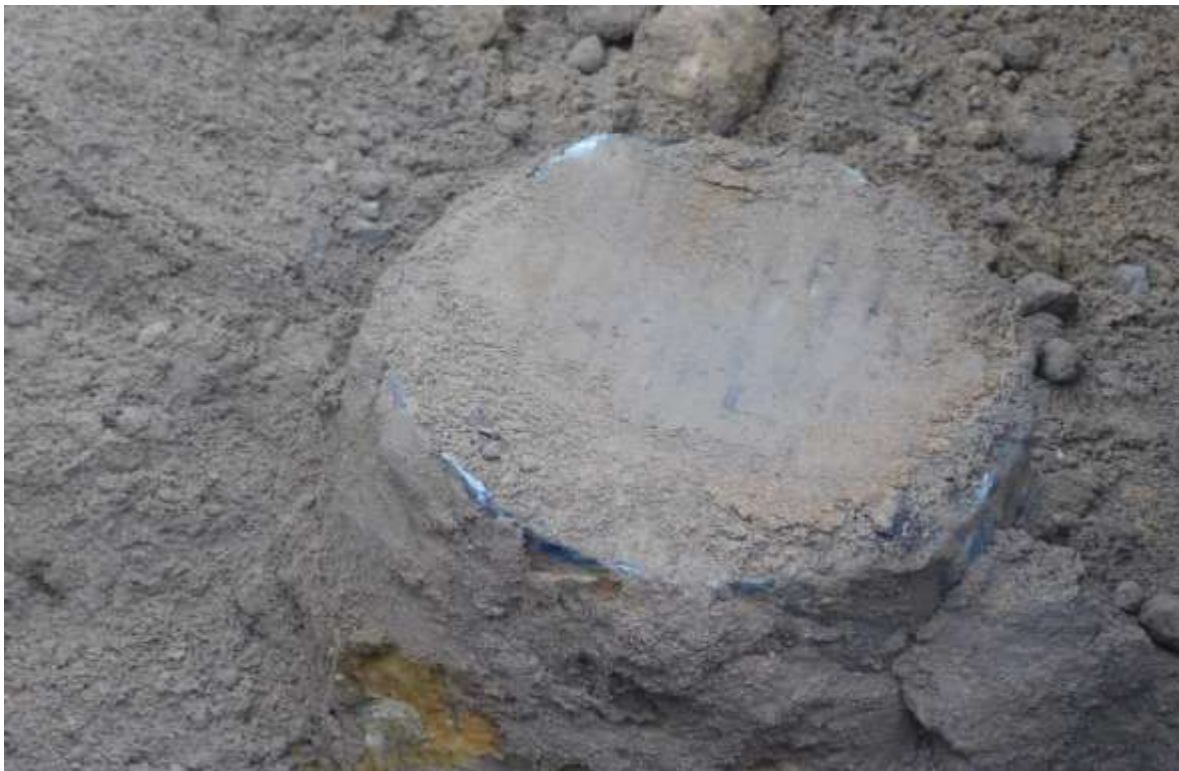
8. Close-up photo of exposed top of well casing in excavation pit.
