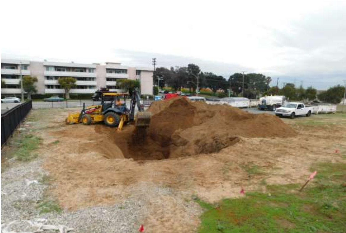
14. Looking north at backfilling of excavation pit after leak testing.
