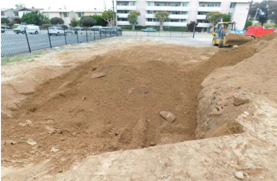
16. Looking north at excavation pit backfilling process.
