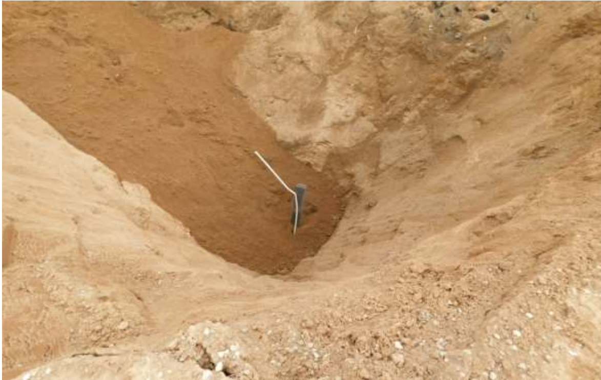
15. Looking east, down into excavation pit during backfilling – marked well casing location with 4 in. x 4 in. x 4 ft. long timber and 10 ft. PVC pipe section.
