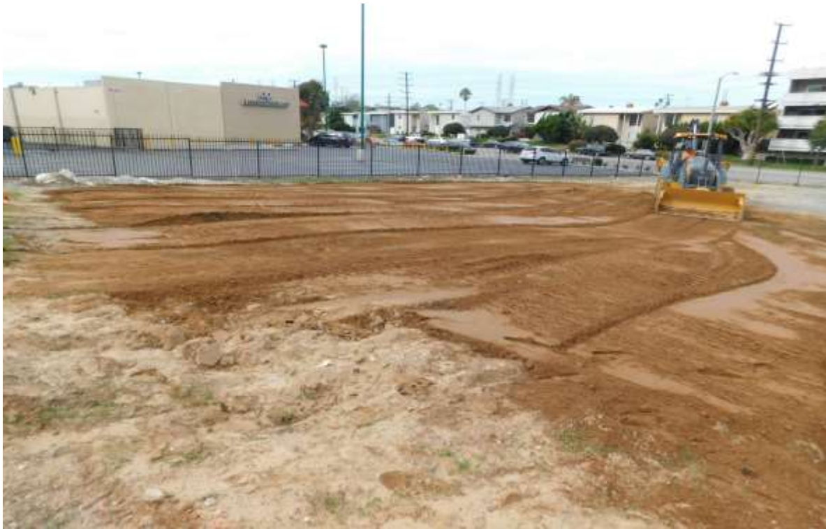
19. Looking west at final excavation pit backfill process, restoring surface grade elevation.
