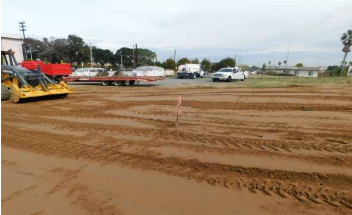
21. Looking east at surface staked location of well casing after backfilling activities.
